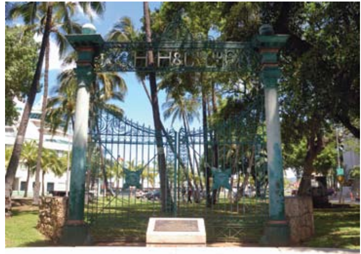
The site of the 1851 court house has been commemorated in Walker Park, next to the Topa Towers on the corner of Nimitz and Bethel. This gate that connected the courthouse with the 1902 Amfac Building has been preserved and is bordered by two short pillars made from courthouse coral blocks, "cousins" to the blocks at MHM.
